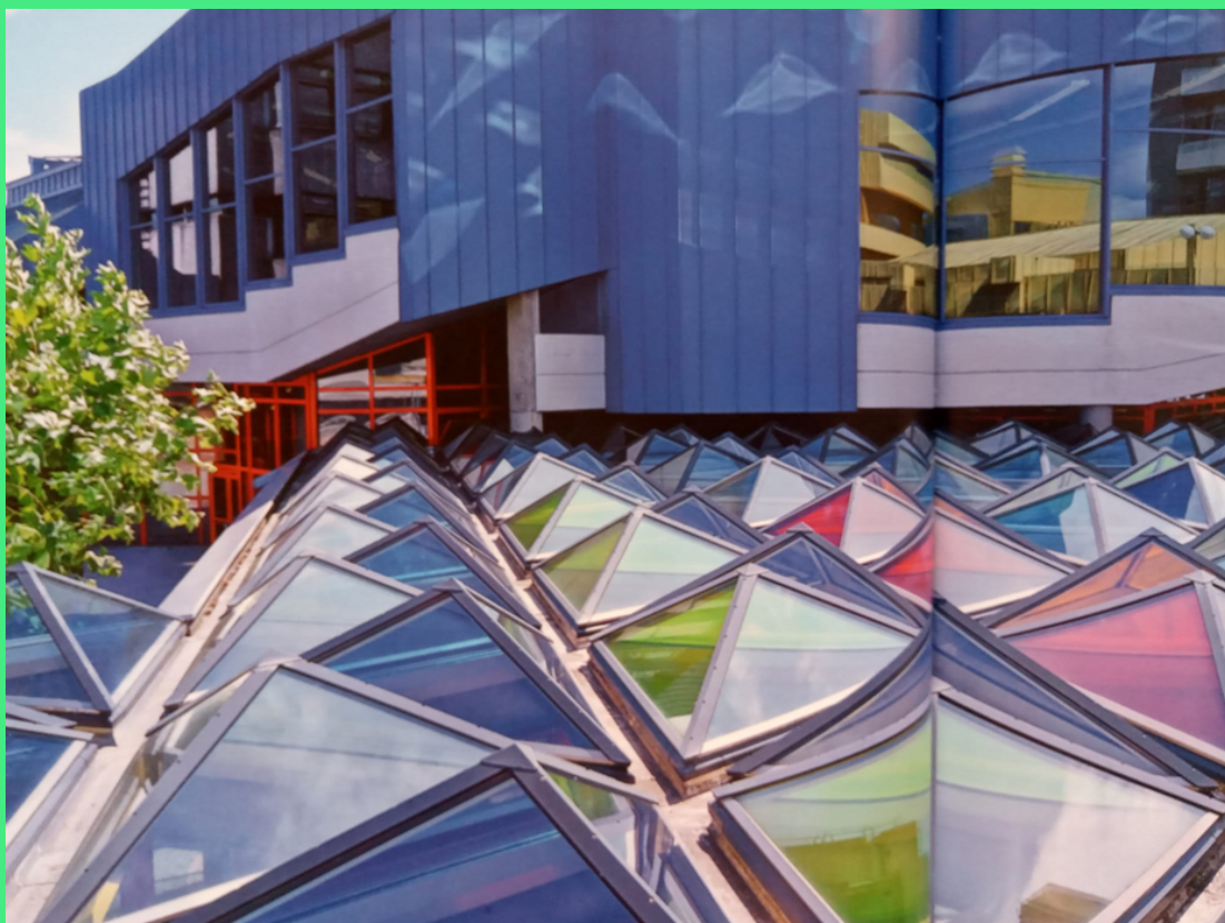
Figure 2: Glass roof over part of the inner courtyard (Reiter, Fotos der Universität Konstanz, 2016.)
